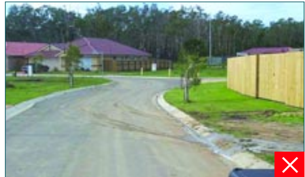
Mud and dirt which has been tracked out onto road
