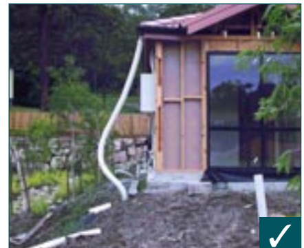
Temporary roof water connection
