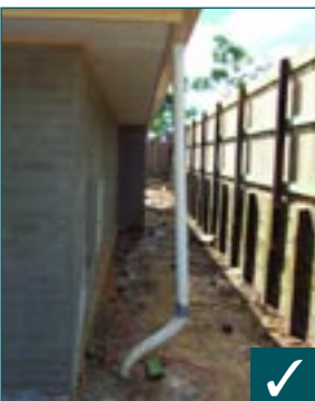
Temporary roof water connection
