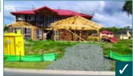
Stabilised gravel entry/exit point (rumble pad)
