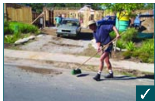
Undertake regular site clean-ups
