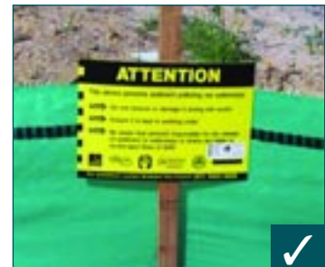
Sediment control information signage
