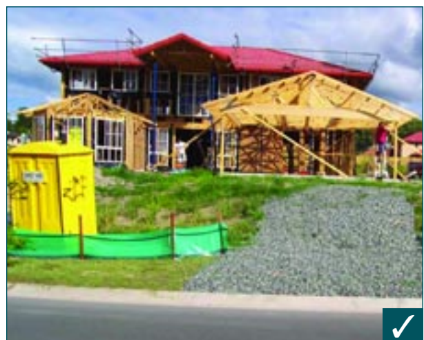
Control measures in place on a residential building site
