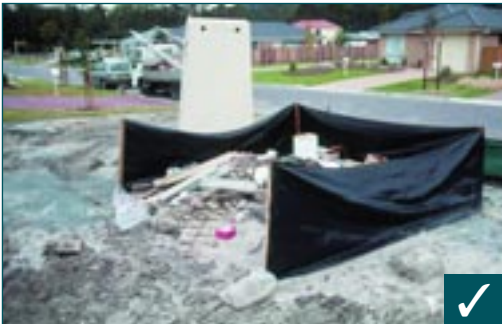
One way to properly store litter and building waste
